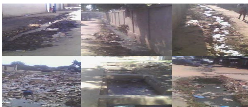
Figure 3. The gutters of N'Djamena mouths by household garbage.
