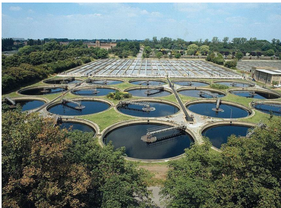
Figure 8. Green Belt around the Waste Water Treatment.
